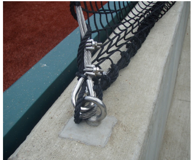
Figure 5. Bottom Cable Termination
