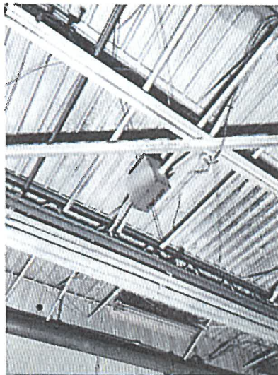
Unsupported Junction Box
